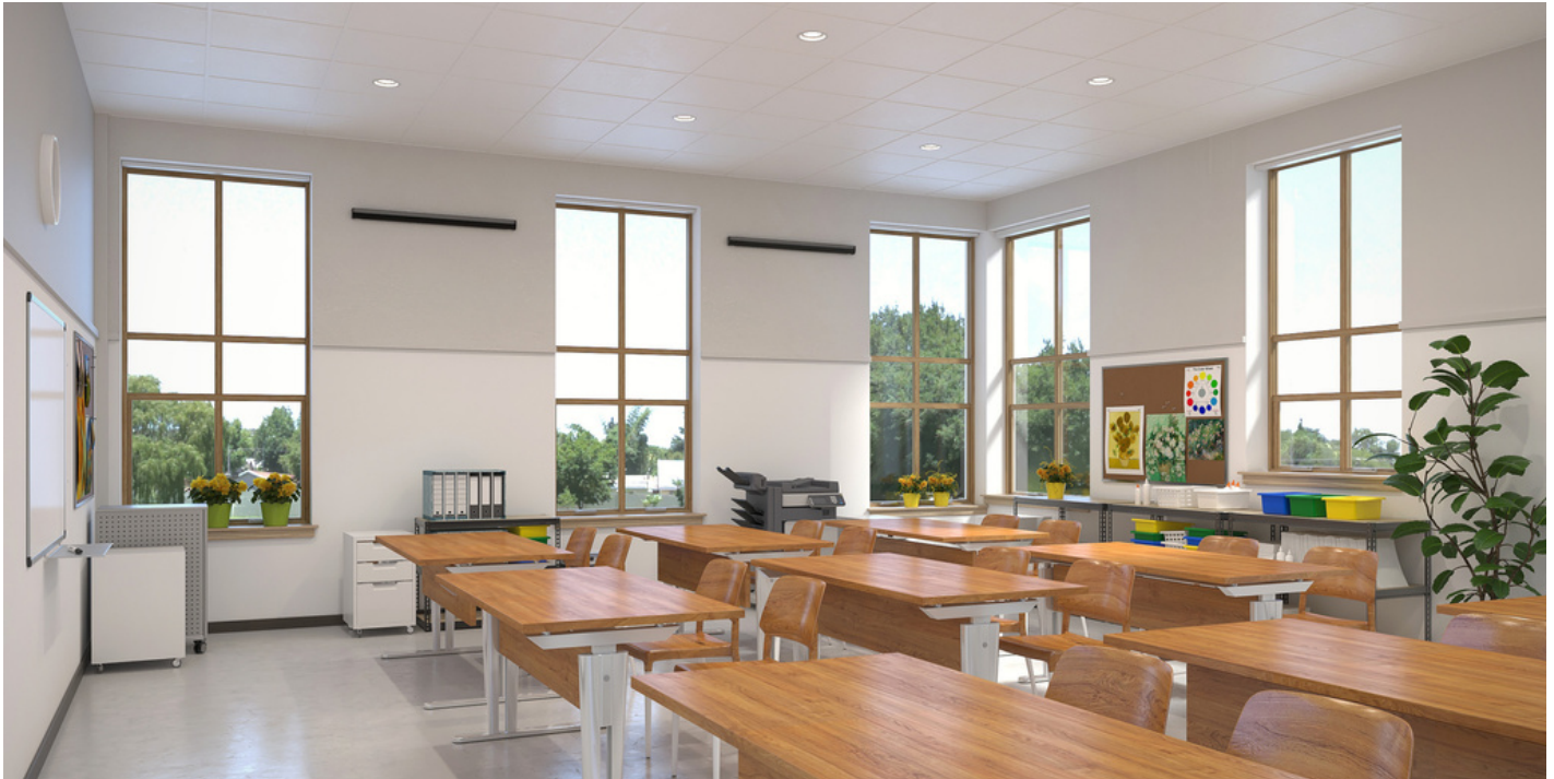
Figure 14: Purifii AER W installed in a K-12 classroom.
