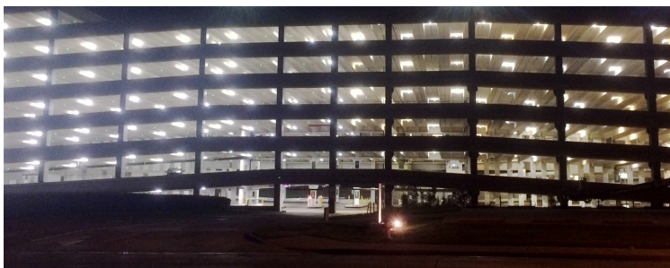
Retrofitted garage on left. Previous lighting system on right.
